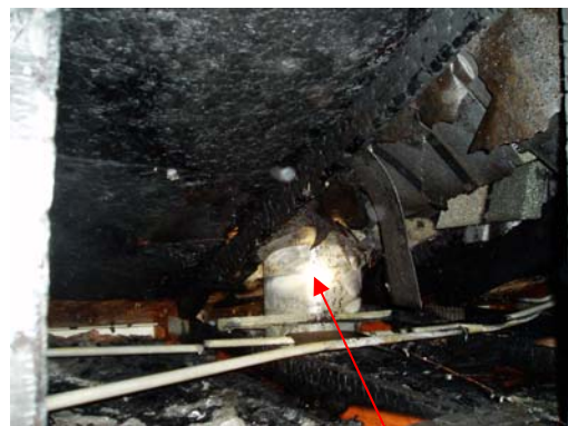
Chimney flue inside attic
