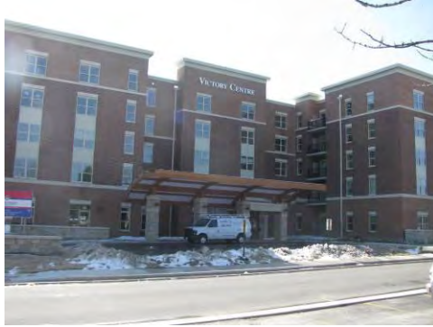
New – Victory Centre Senior Apartments & Supportive Living 97 & 99 Phillip Dr. – 182,061 sq ft 231 Units
