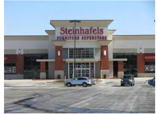
Remodeled – Steinhafels Furniture 569 Milwaukee Ave – 102,625 sq ft
