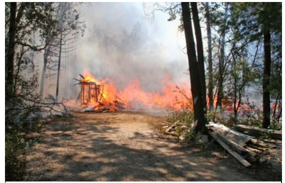
Fire Origin – Single family home under construction.
