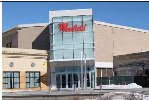
New – Southwest Mall Entrance - Remodeled
